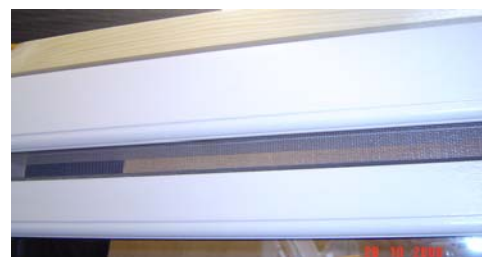
2 – Top sash partially open, you can see the screen is attached to the top of the top sash
